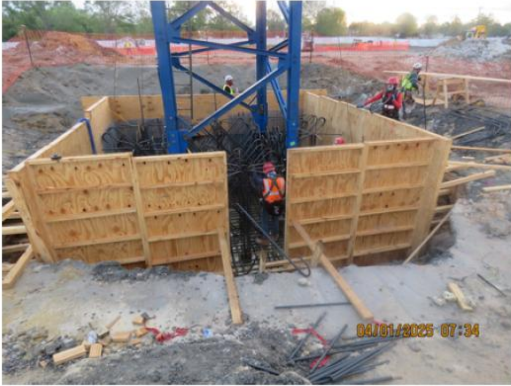
Tower Crane Base Barrier
