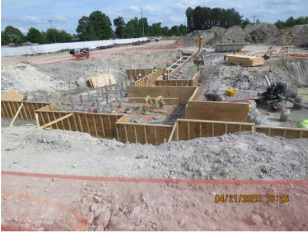
Forming Mat Foundation at Stair 4 & Loading Dock
