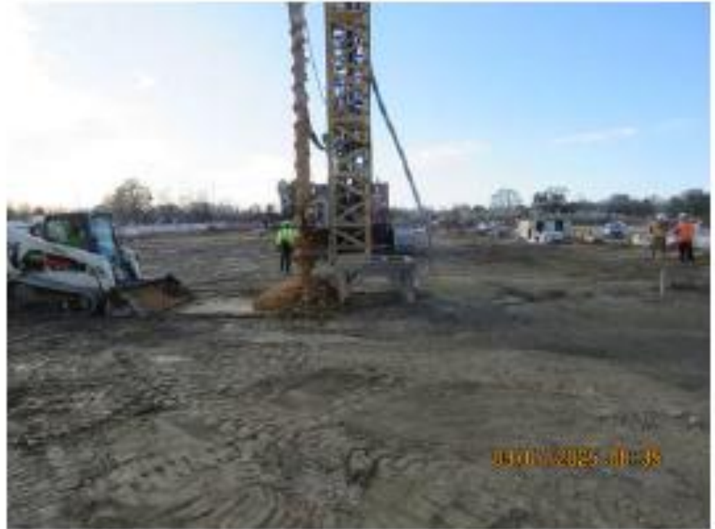
Keller Continuing with Case Piles
