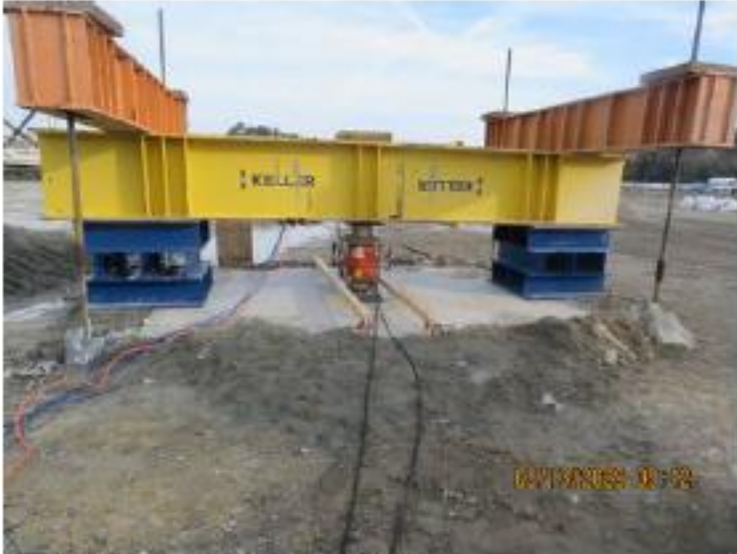
Test Pile Rig for Keller Test Piles
