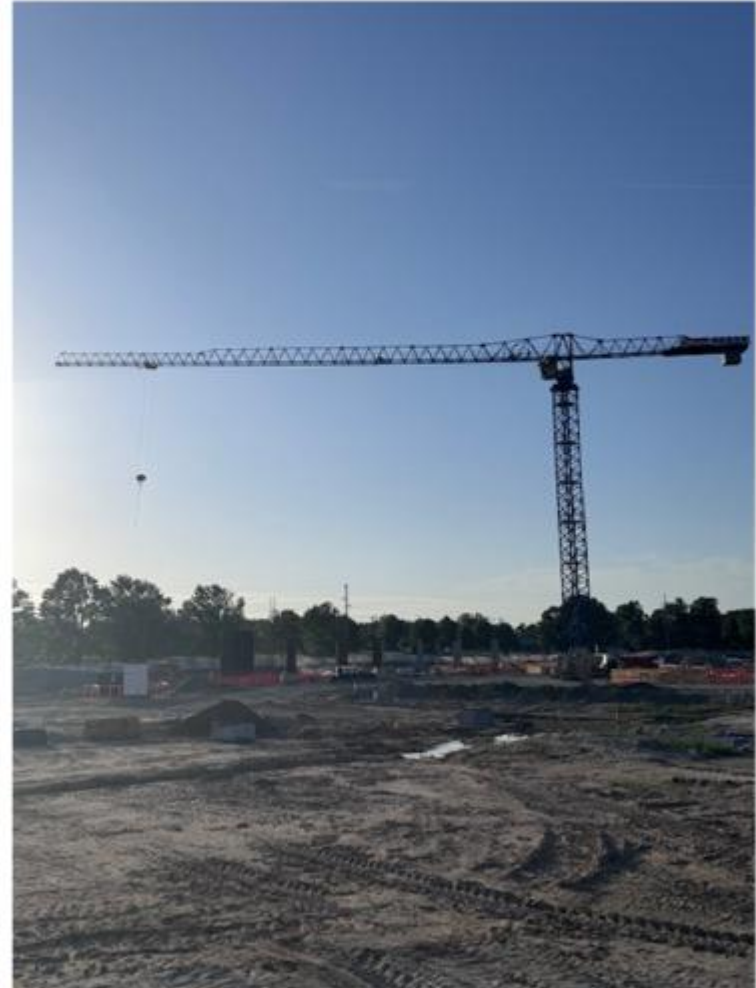
Tower Crane Erected & Operating at Full Capacity
