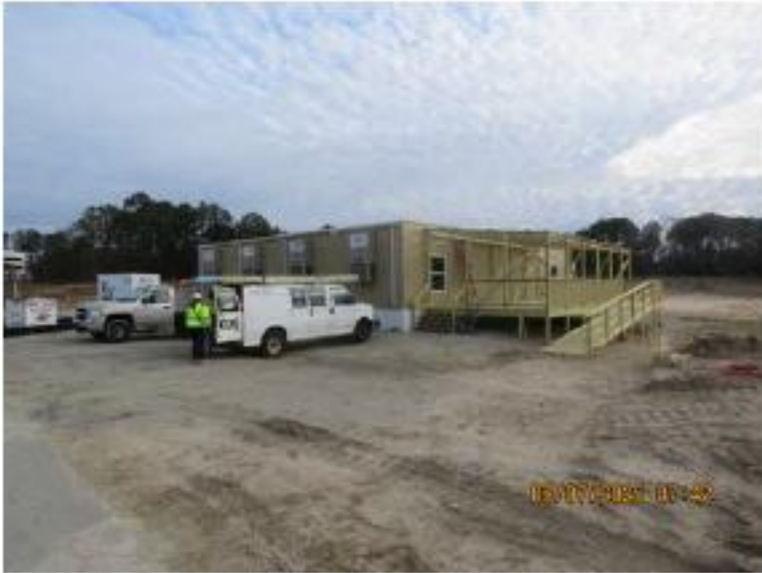
Gilbane Trailer and Deck Being Installed
